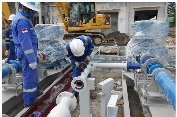
(Piping & Pump Intallation)
