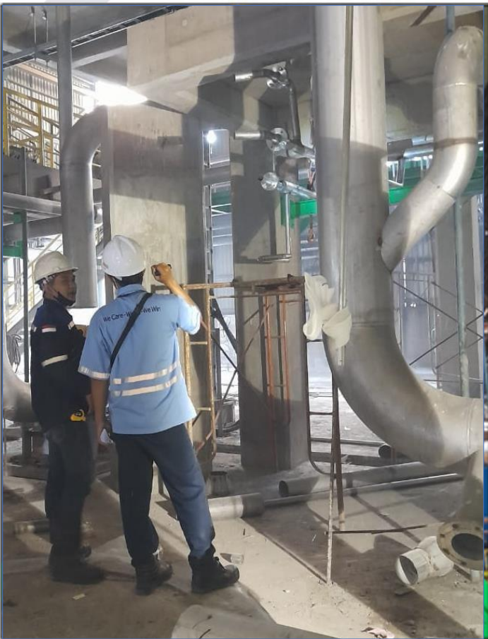
(QC Inspeksi After Instalation)
