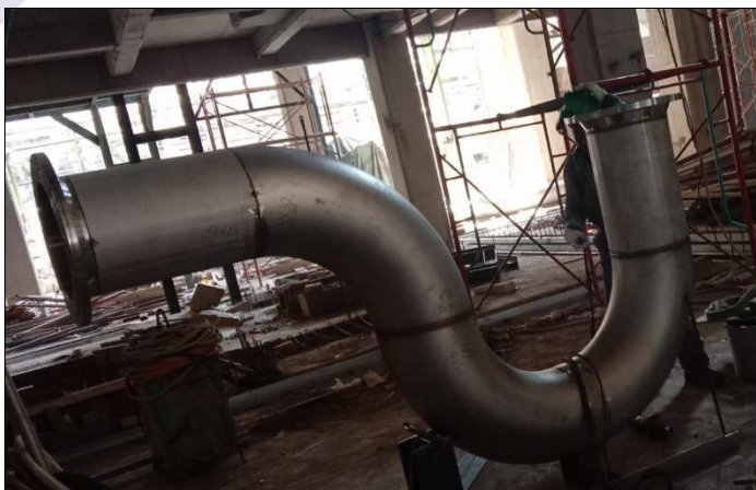
(Process Piping Installation)
