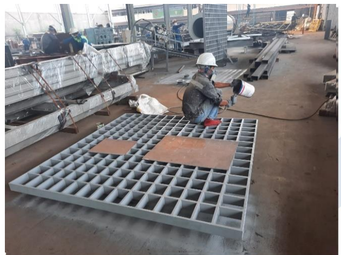
(Screen Hopper Fabrication coal UNIT PLTU)
