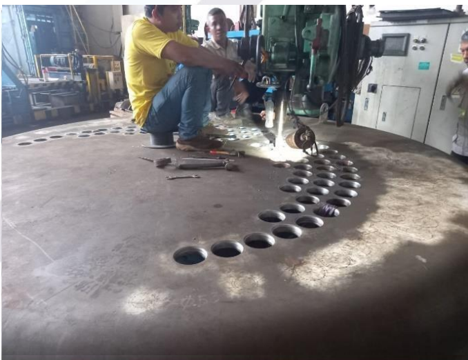
(Tube Sheet Boiler Drilling Process)
