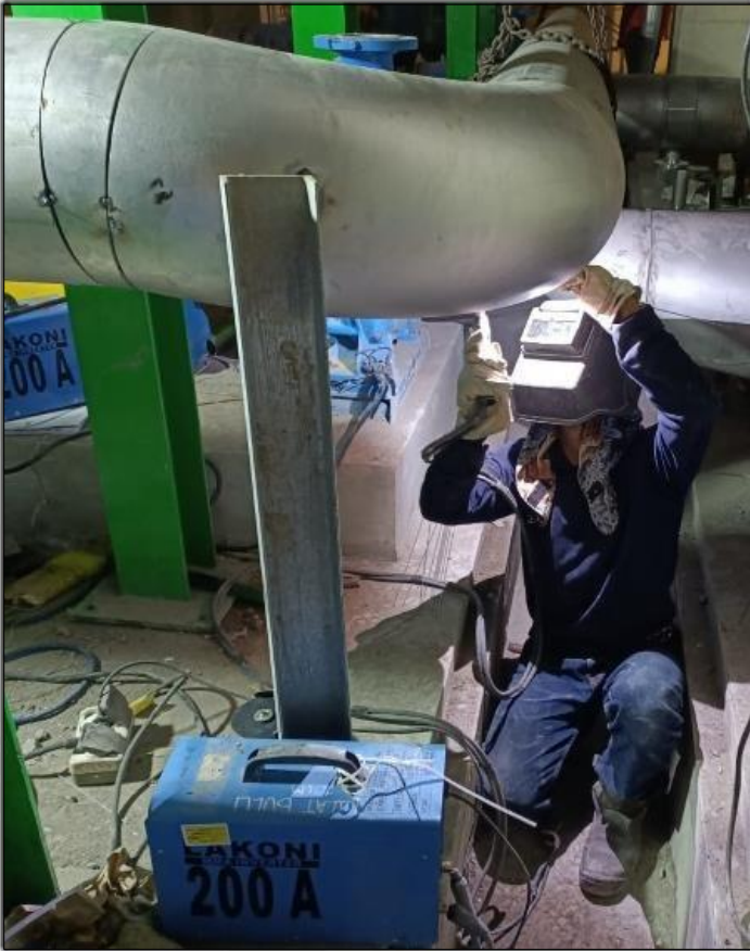
( Piping & Welding Installation )
